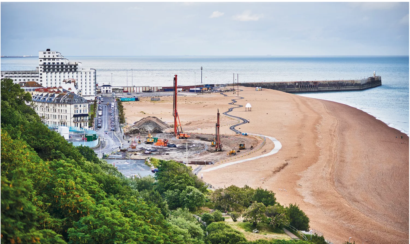
The 200-plus continuous flight auger (CFA) piles are around 30m deep (Photograph: Matt Rowe)
